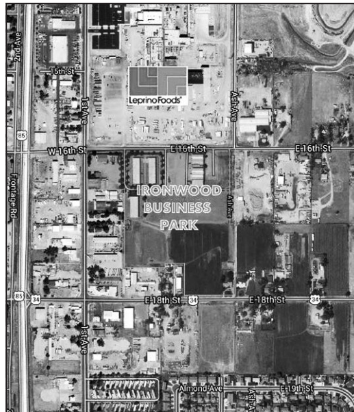
New development is planned for Ironwood Business Park in Greeley.
